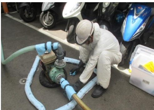
Conduct checkpoints for chemical tanker loading
