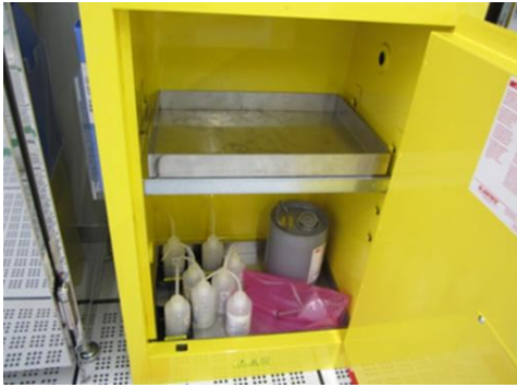
Chemicals storage cabin set up with leak prevention tray
